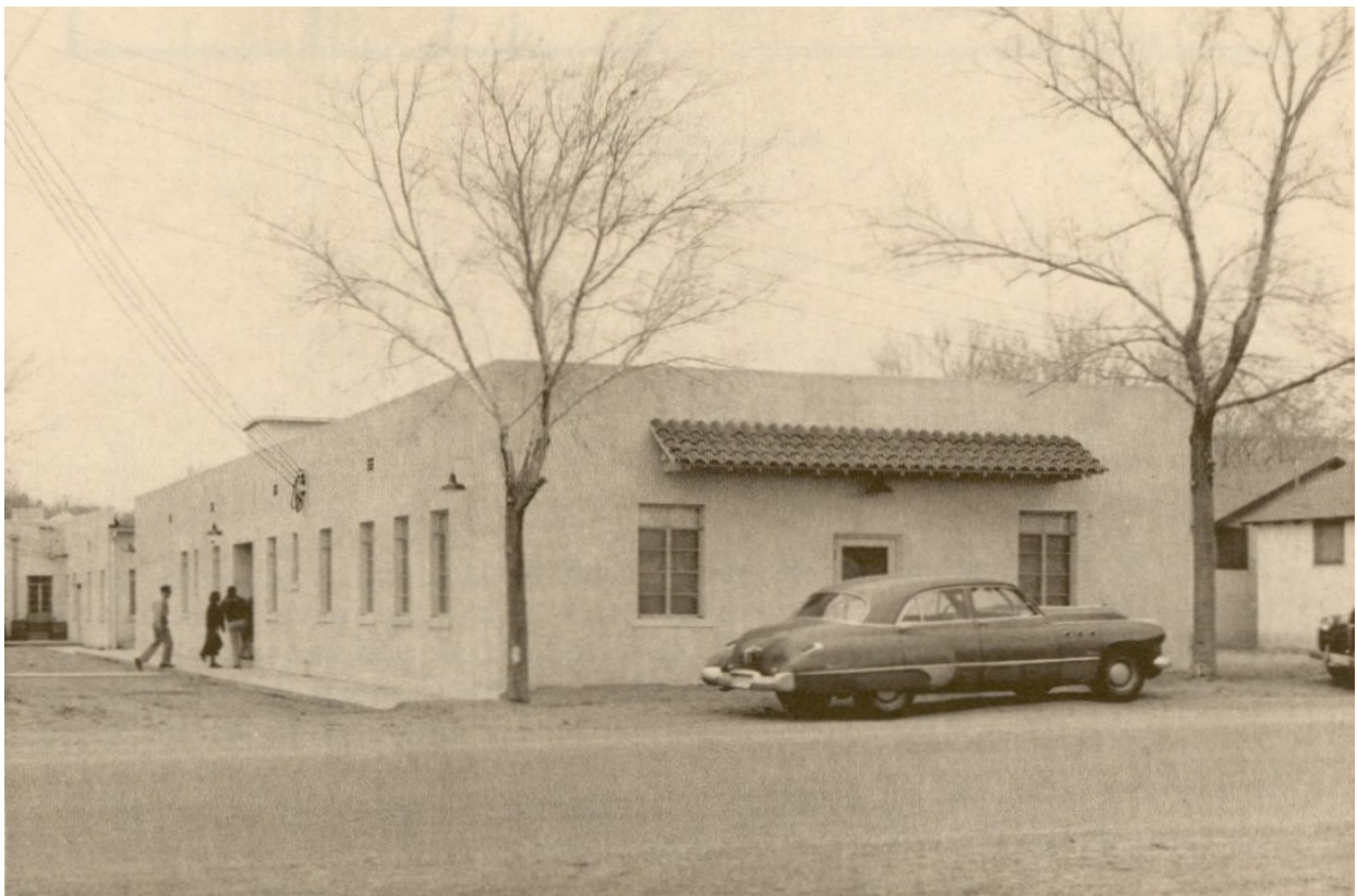
Figure 39. PSL Building Annex, South View, 1953
