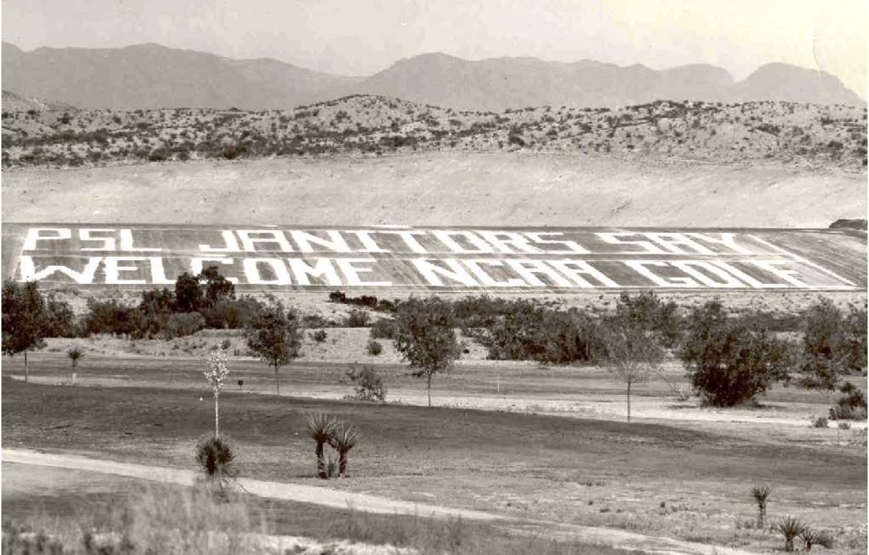
Figure 93. Original Layout of the “Welcome NCAA Golf Tourney” Message on the Flood-Control Dam Spillway, Spring, 1968
