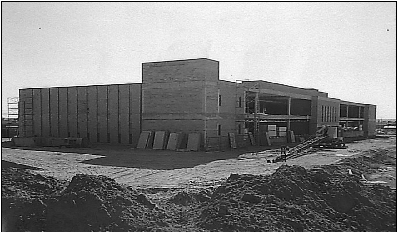
Figure 90. The "Shell" Nears Completion, 1964
