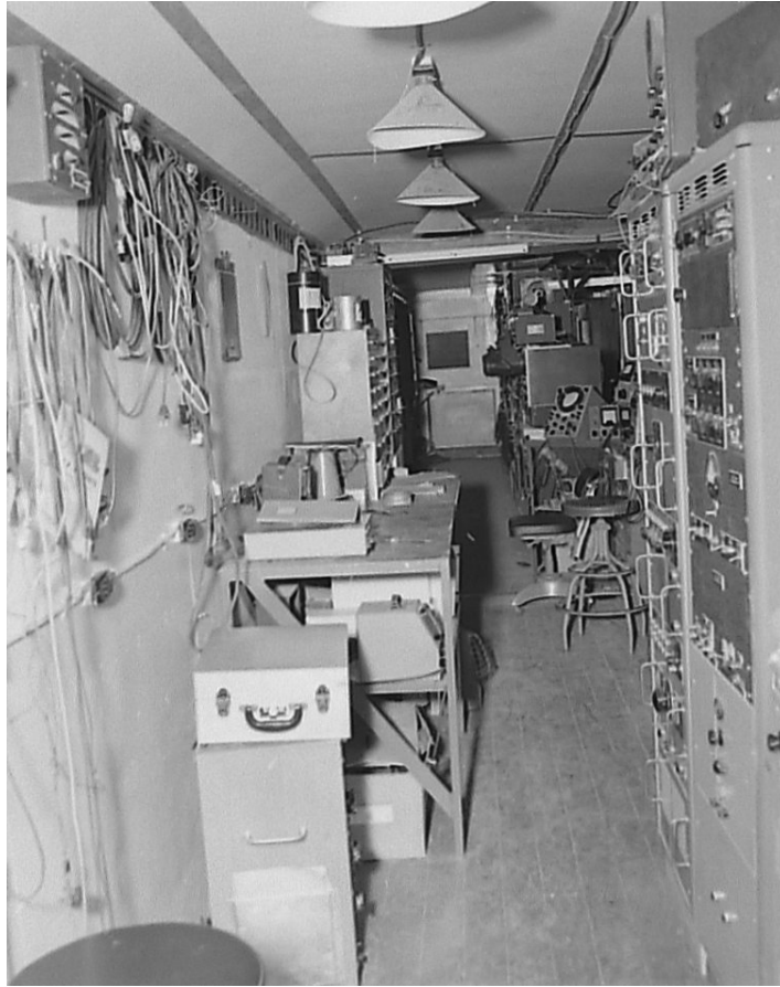
Figure 36. Interior of the Red Wagon
