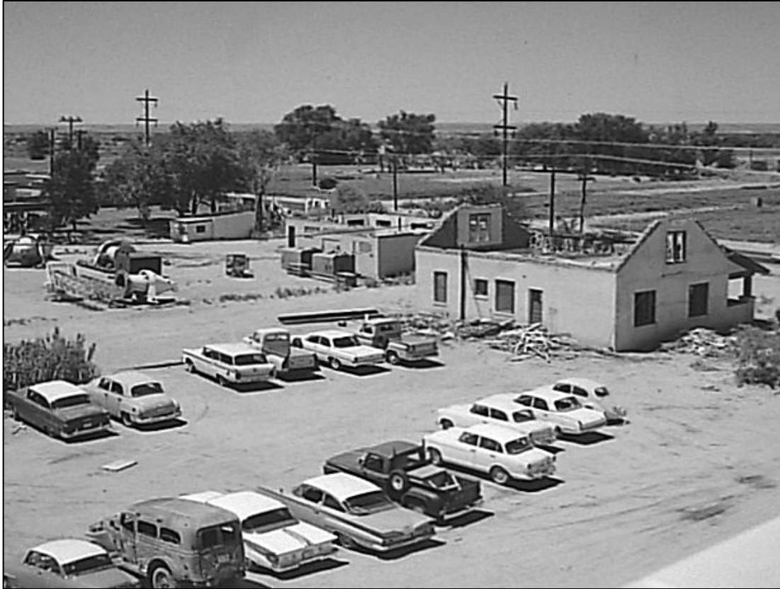
Figure 117. Demolition of Old Houses for Construction of PSL's West Parking Lot
