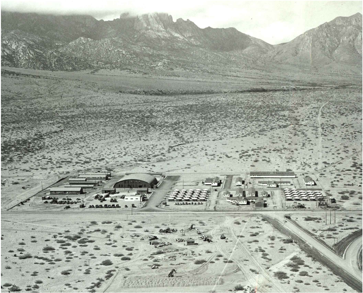
Figure 8. WSPG Headquarters and Support Buildings, 1946
