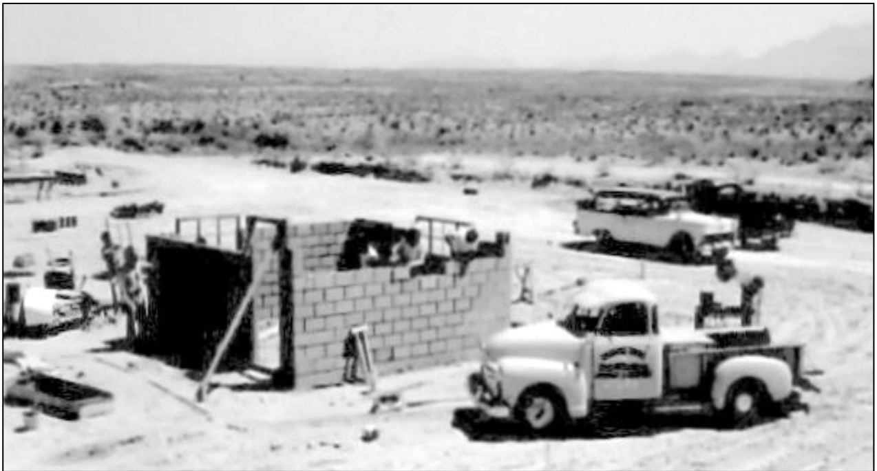
Figure 98. Antenna Range under Construction
