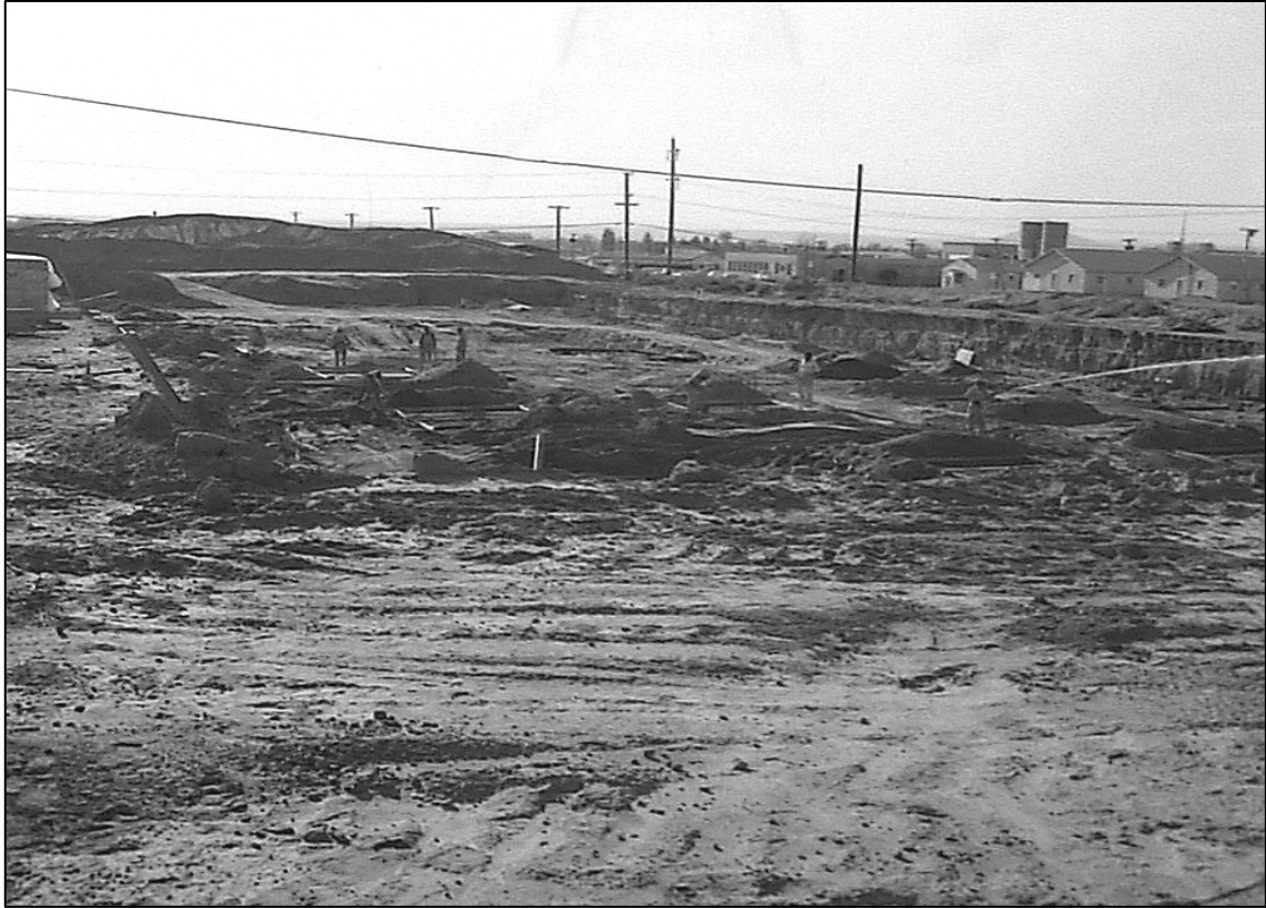
Figure 89. Excavation for PSL Building, 1963 looking to the NW (notice barracks)
